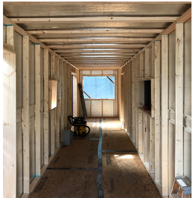
Figure 2. Interior framing over polyiso. Photo by author.
